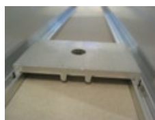
Fastening between the collectors.
